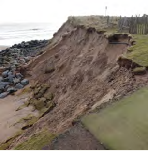
Erosion at Montrose
